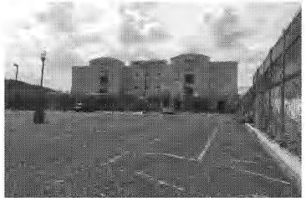
View of ARC exterior and parking lot to west
