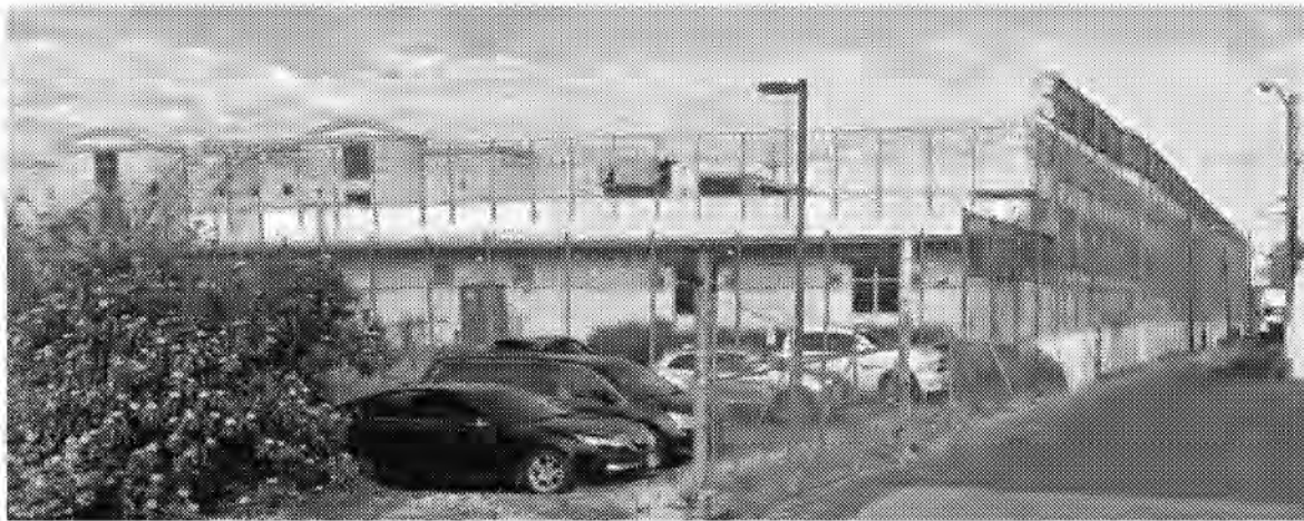
Converted 1963 Warehouse at 377 Enterprise Avenue, facing northwest
