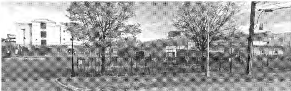
ARC Buildings at 375-377 Enterprise Avenue, facing north/northwest
