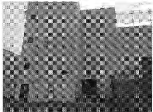
View of ARC towards south
