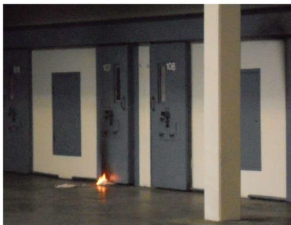
Fire set by a prisoner in a solitary confinement unit, East Mississippi Correctional Facility, April 3, 2014
