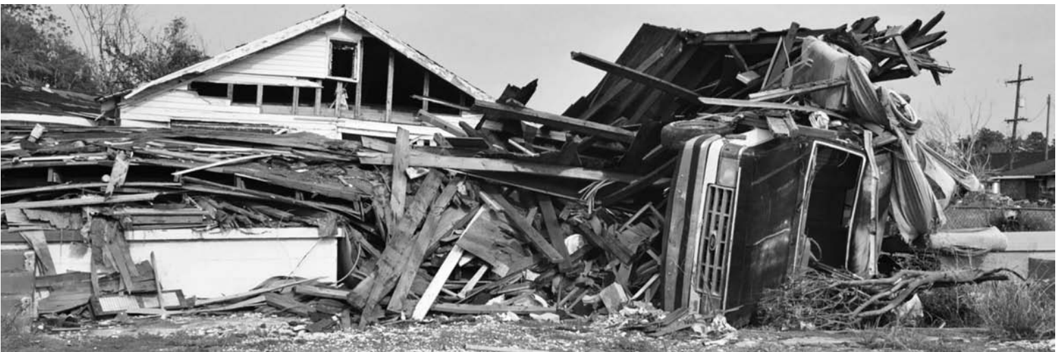
Destruction like this was common in New Orleans after Hurricane Katrina.
