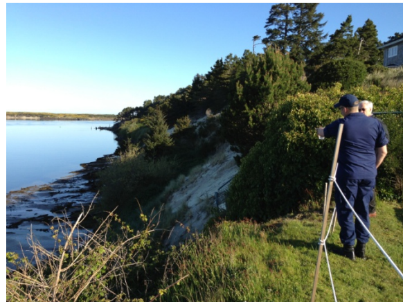
Erosion at Station Siuslaw
