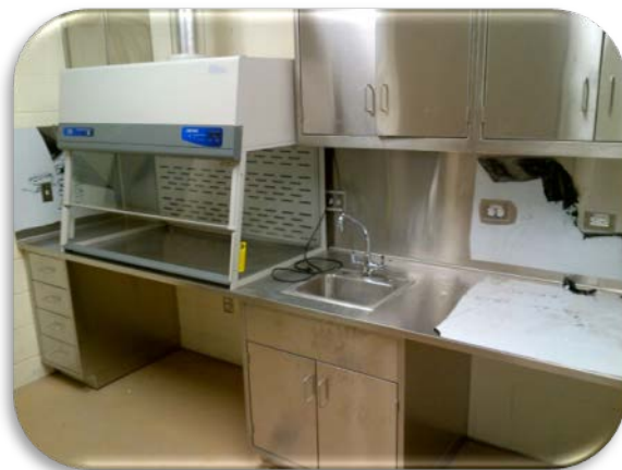
Exhibit 3. New agriculture laboratory being installed with fume hood (to mix chemicals) to the left of the sink.
