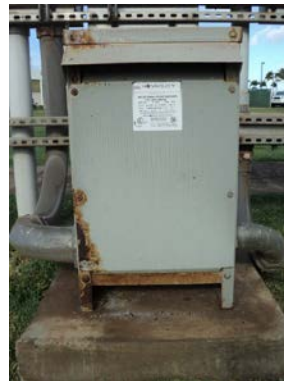
Corroded Transformer
