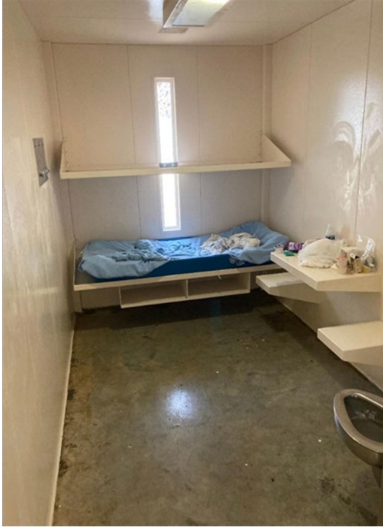
Figure 1. Photograph of a cell at the SC DJJ Juvenile Detention Center (taken by the author on August 7, 2020).
