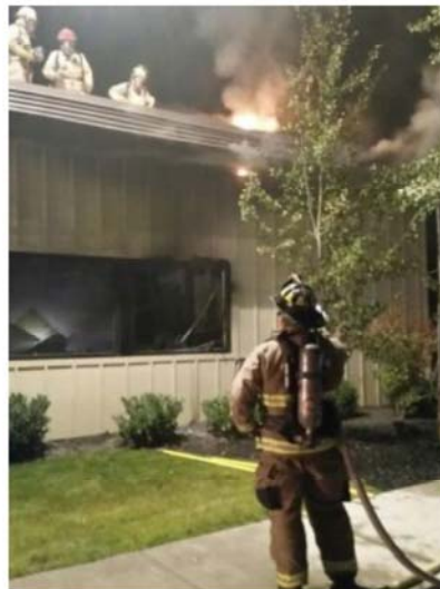
(U) Firefighters respond to a September 2015 arson of a Planned Parenthood USPER facility in Pullman, Washington.
