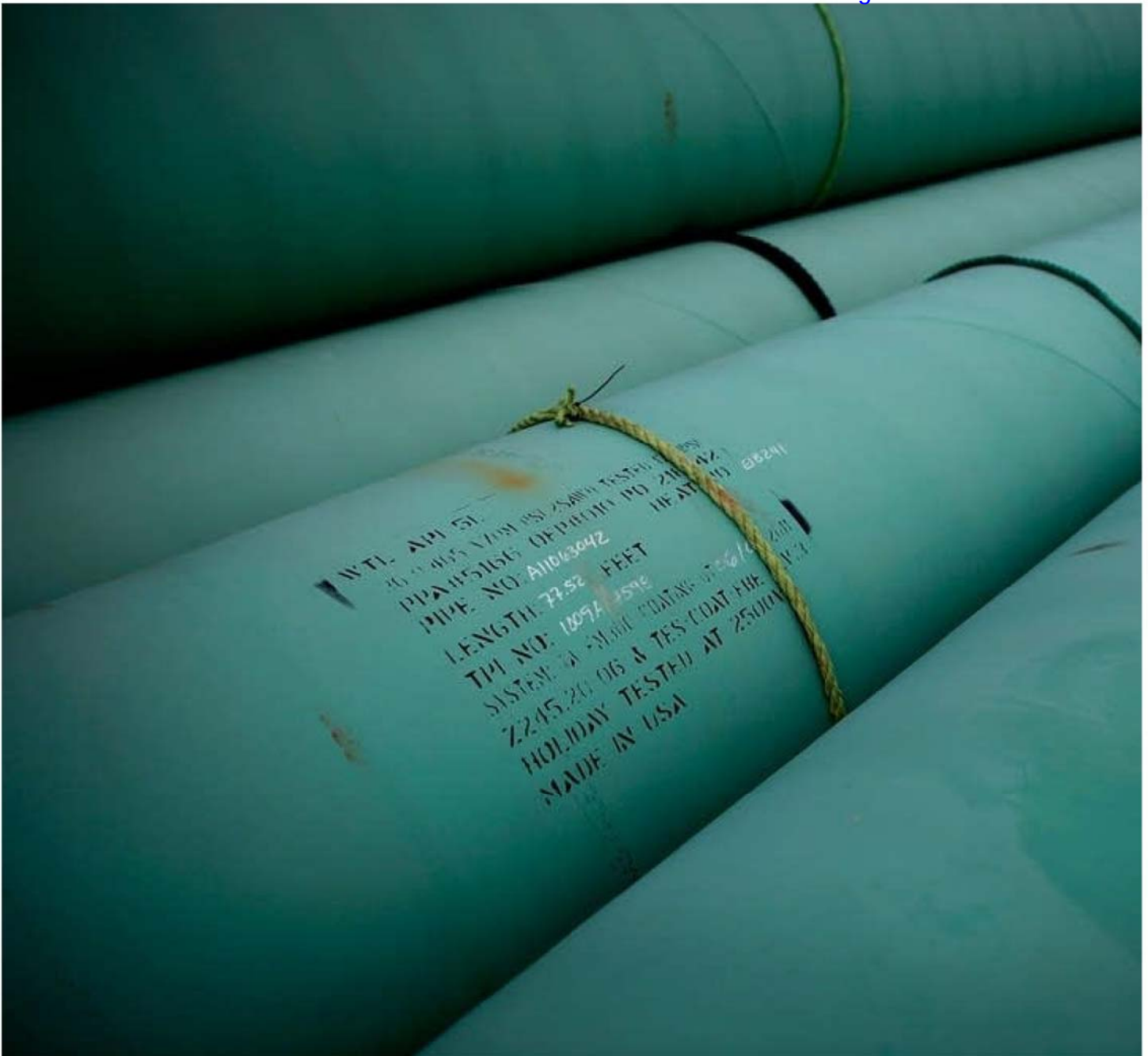
Pipe is stacked at the southern site of the Keystone XL pipeline. Tom Pennington | Getty Images 2012
