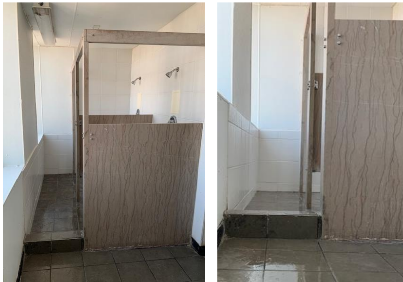
(Photographs 129-130, Infirmary 4th Floor Shower Behind Nurse's Station).
