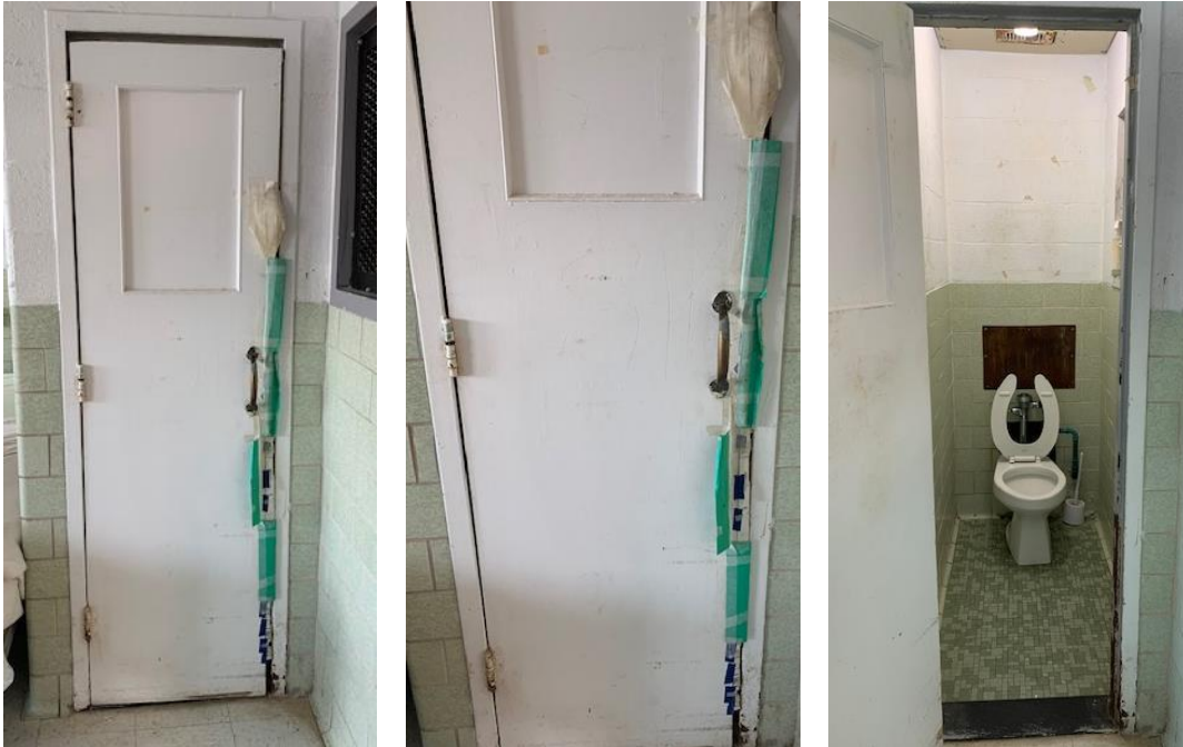
(Photographs 155-157, Room 309 Toilet)
