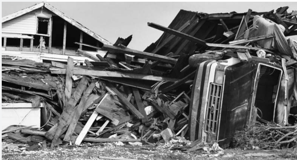
Destruction like this was common in New Orleans after Hurricane Katrina.
